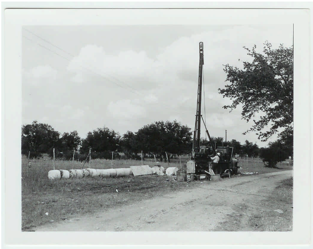
Figure 2. View of the auger rig of the Texas Highway Department District 14 and driller, Jim Cole, when the two-foot access hole to cavern below had been completed (photo taken by Jack Lewis, photographer with the Travel and Information Division of the Texas Highway Department, 1963).
