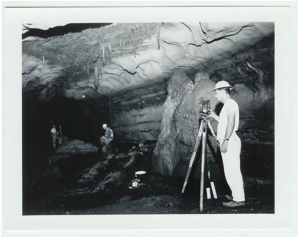
Figure 4. Survey crew working inside the Discovery Room with Leroy Sumner operating the survey instrument, Bill Johnson recording survey data, and James Sansom holding survey rod at a distance. Note light on cord hanging down from roof of cavern providing light for surveying (photo taken by Jack Lewis, photographer with the Travel and Information Division of the Texas Highway Department, 1963).
