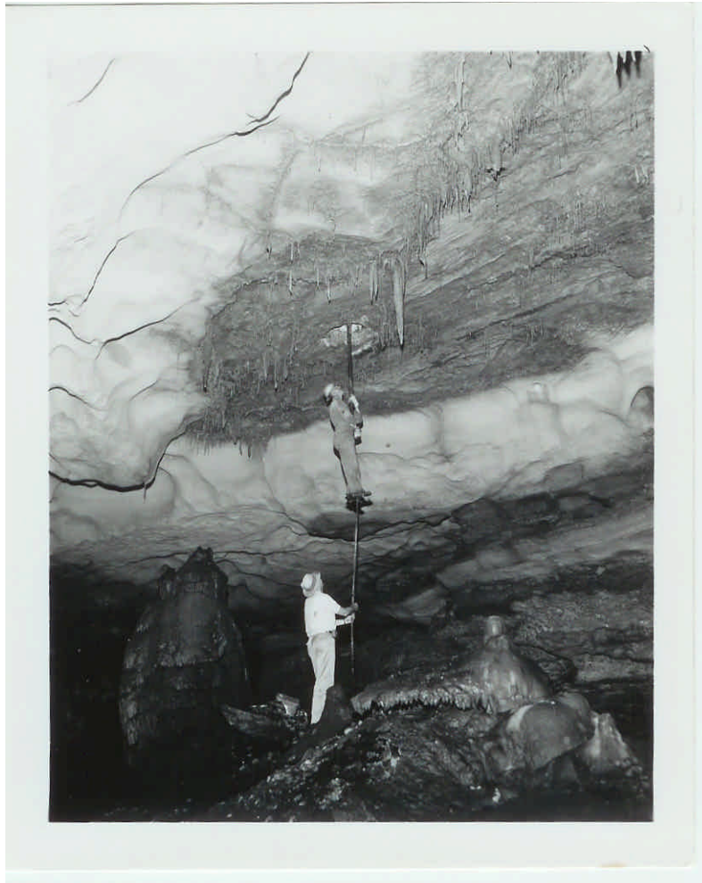
Figure 3. View of the inside of the Discovery Room of the cavern where Bill Johnson, Texas Highway Department Survey Crew Chief, was being lowered into the cavern on the auger rig kelly through the two-foot diameter access hole. James Sansom was holding the guide rope on the kelly (photo taken by Jack Lewis, photographer with the Travel and Information Division of the Texas Highway Department, 1963).
